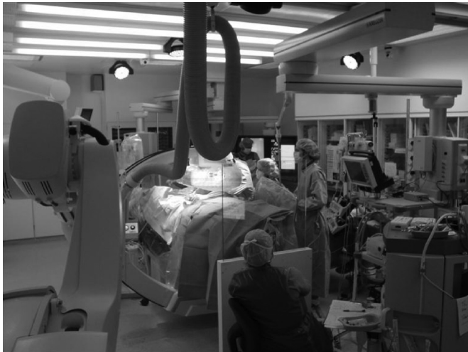
Figure 4. Set-up of a hybrid operating room at Rikshospitalet in Oslo, Norway. The robotic multi-axis system offers high flexibility and advanced 3D imaging capabilities in the operating theatre. Convenient park positions maximize space in the room and keep the system out of the way when not needed. Courtesy of Professor Fosse, Rikshospitalet, Oslo, Norway.
